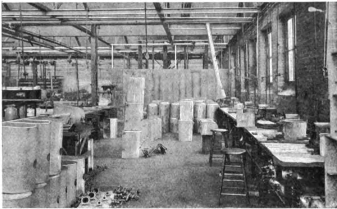
SPACIOUS ROOM WHERE THE TANKS ARE MANUFACTURED.
